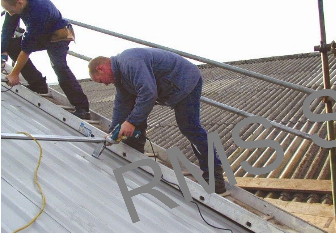
Working above ground level
